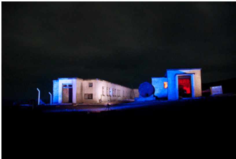
Former Listening Station, Garthsness, South Mainland, photographed by Austin Taylor
